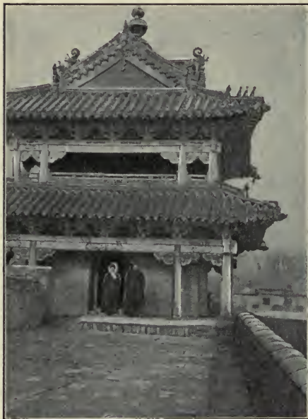
Tower at Shanhaikwan.
